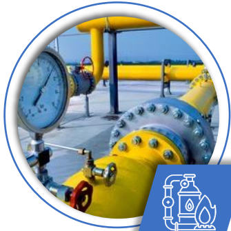
City Gas Distribution
